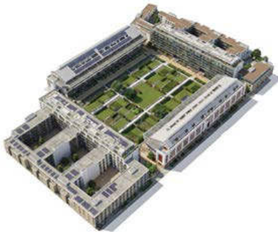
Leisure facilities: Former Highbury Stadium, Highbury Square
