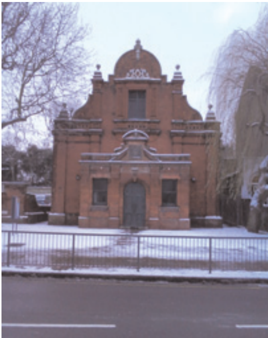
Charlton House estate: 19C Charlton Village Assembly Rooms, built for the community by the Maryon Wilson family, the last residents of Charlton House. The Council intended to turn the site into a car park and the Society initiated a campaign to save and restore it; now Grade II listed
