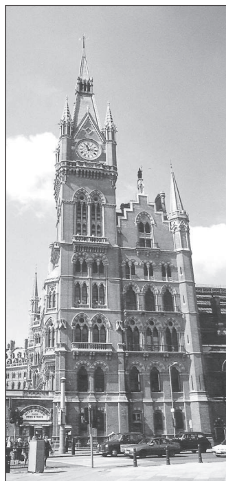
St. Pancras Station -the iconic hotel frontage
